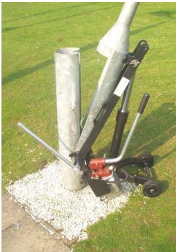
3. Open the control valve to start lowering
